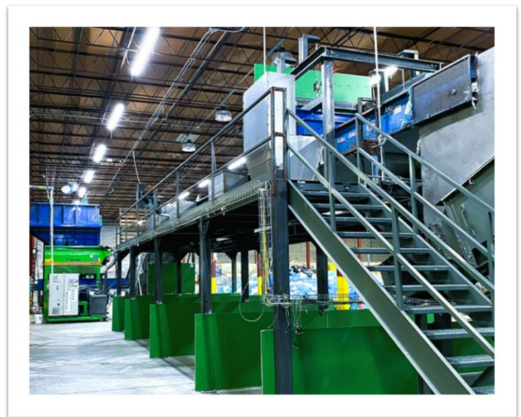
Figure 7. Nexus Circular recycling facility.
